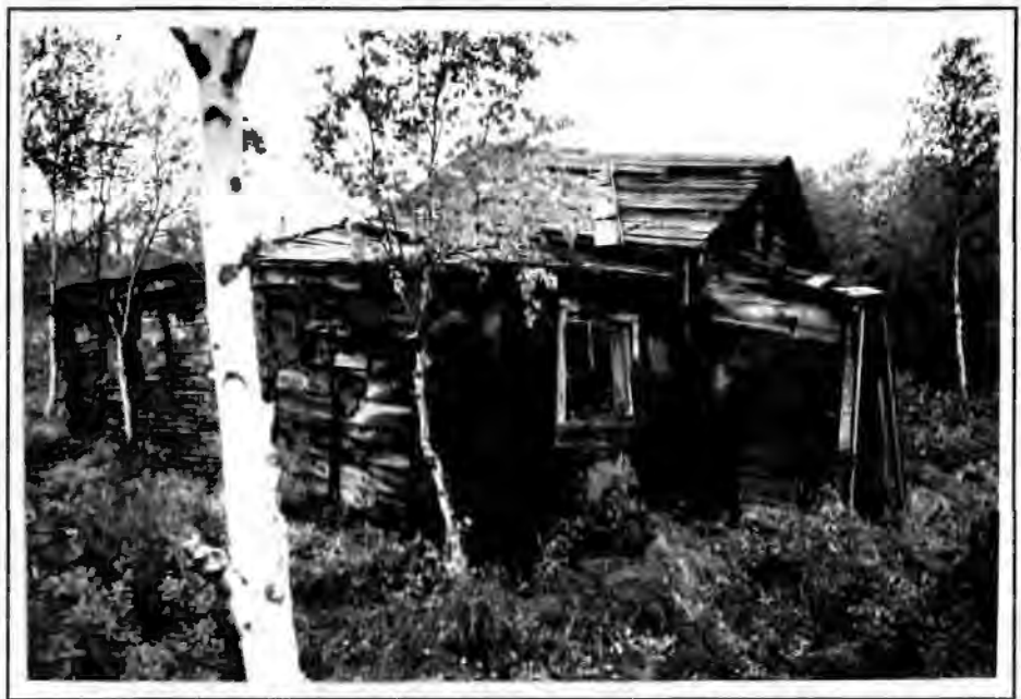
Figure 86. The Crook/Caughrean/Demientieff House, 1993. The view is looking northwest.
